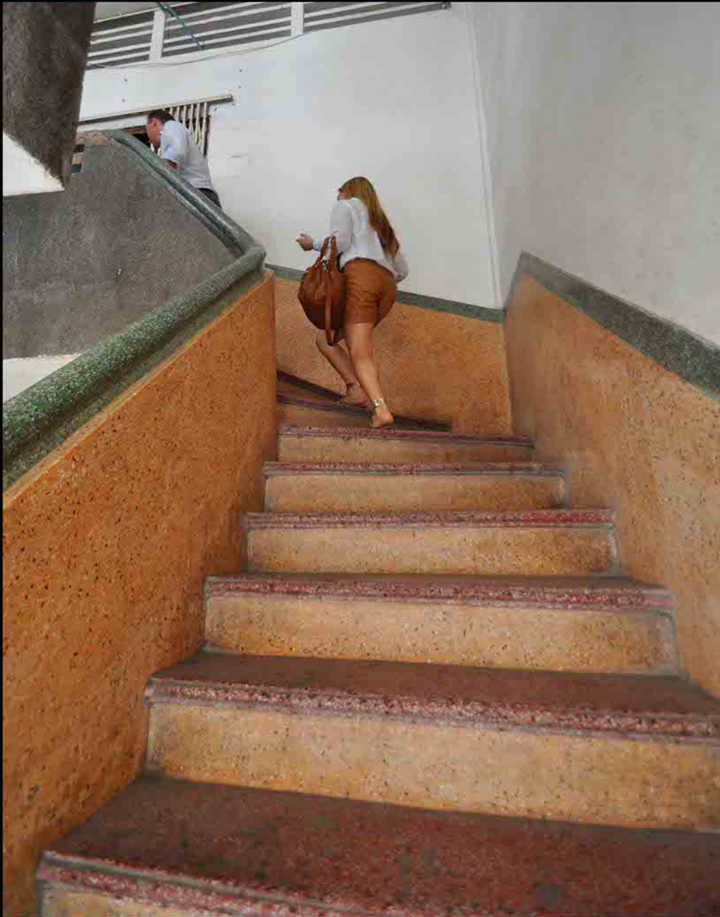
Staircase from main entrance to apartments on first floor
